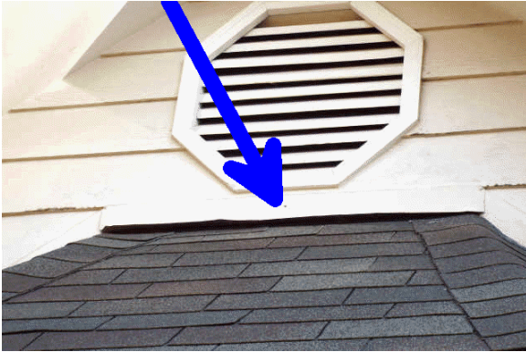
The roof/wall flashing is loose on the front.
