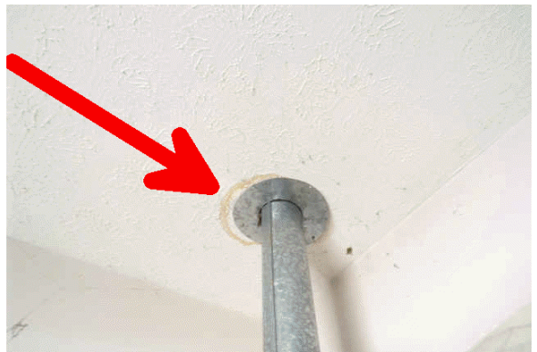
Water stain noted at the water heater flue.
