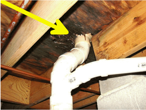
The water damaged subfloor and the cut joist needs to be supported.
