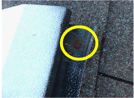
The exposed nail heads at the ridge vent need to be sealed.
