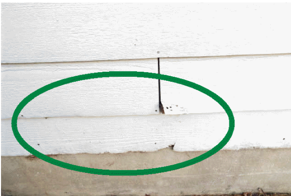
The damaged siding needs to be replaced.
