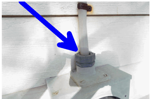
The electrical service cable needs to be caulked. The rusty clamp is staining the siding.
