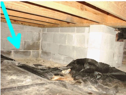
Water stain noted at the front foundation.
