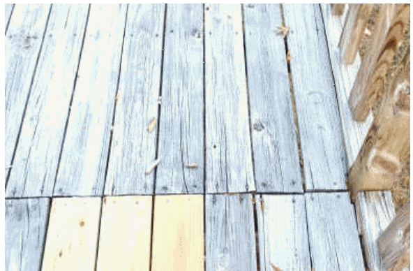
The planks are cracking on the deck.
