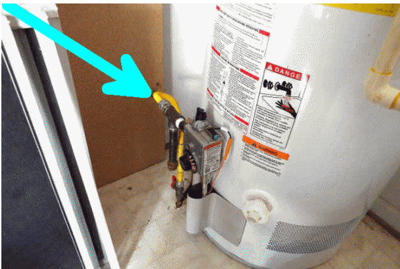
The CSST appliance connector noted at the water heater.
