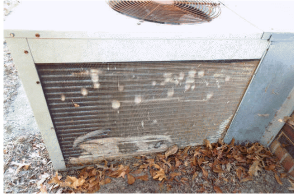
The aluminum fins are bent on the A/C unit.
