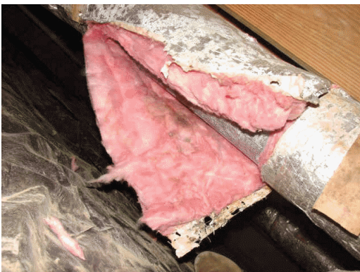
The loose insulation around the A/C duct needs to be replaced.
